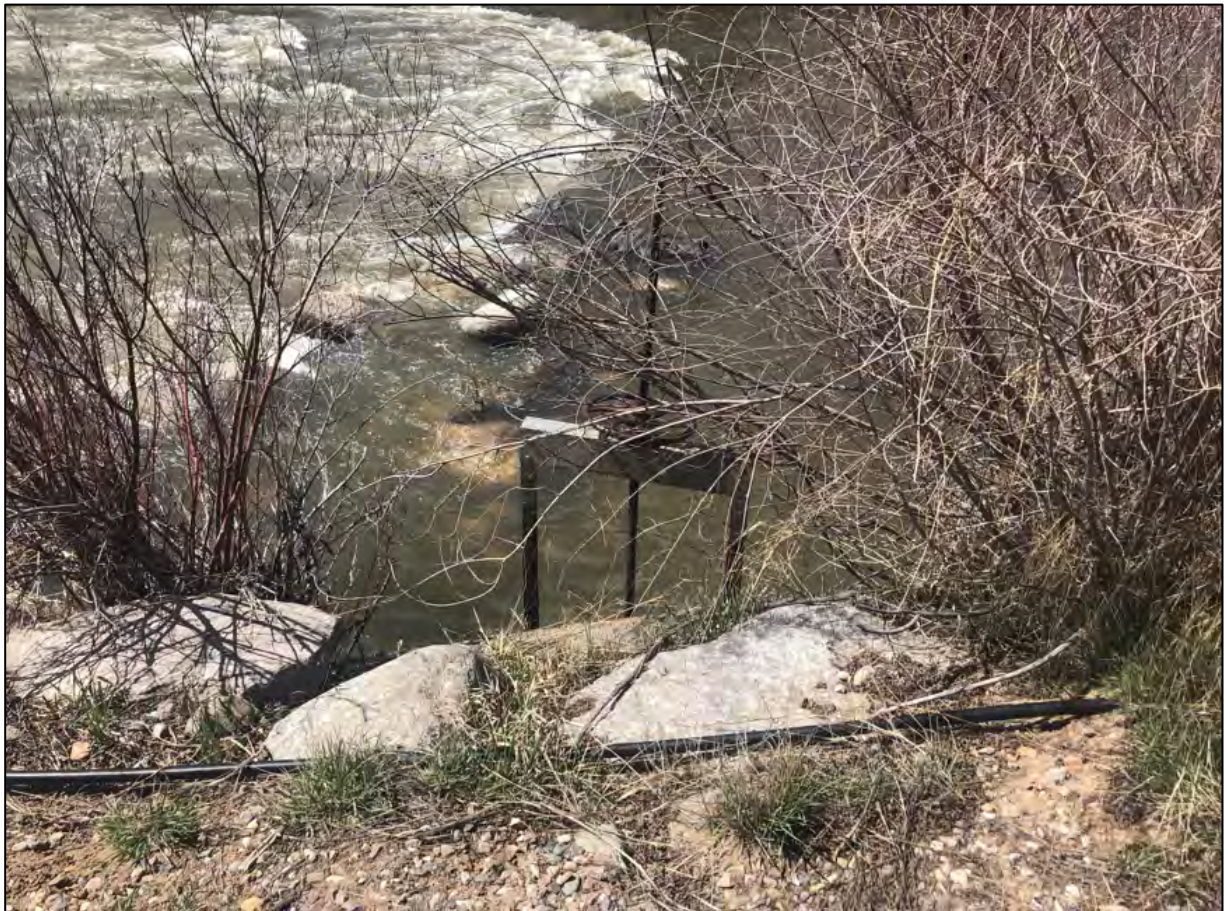
Figure 2-1. Eagle River Intake
